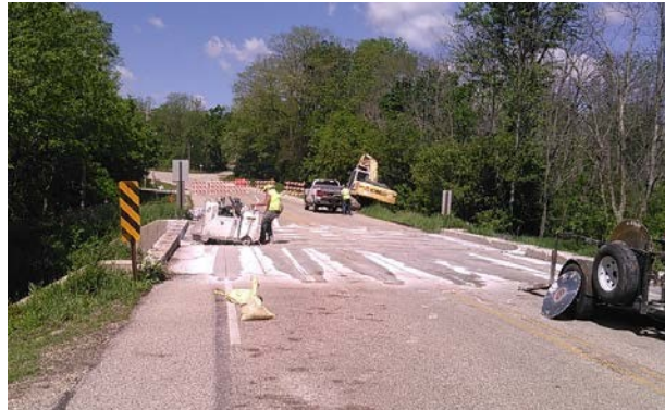
Contractor saw-cutting old deck for removal
