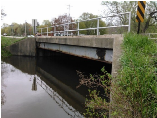
Honey Creek Bridge - Built in the early 1940's
